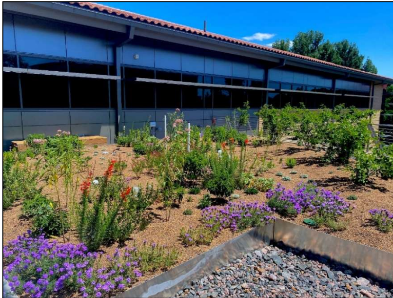
Colorado State University Nutrien building green roof on July 21, 2022. © Kyle Ruskowski
