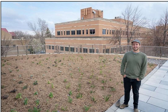
Kyle Ruszkowski stands by the newly planted Colorado State University Nutrien Building green roof on May 3, 2022. © Jennifer Boussetot
