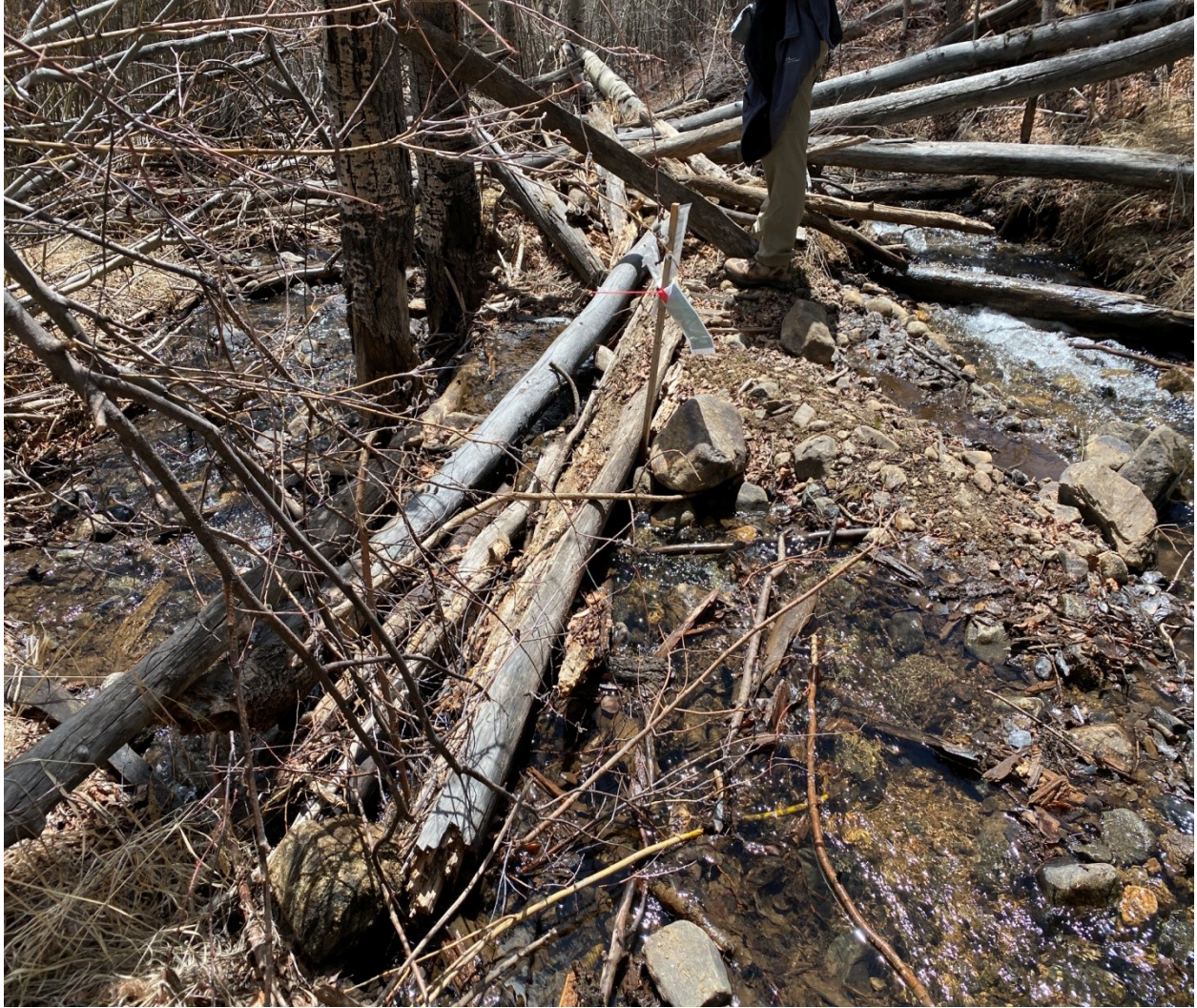
Looking south with east fork on left and west fork on right. Upper DWR partial diversion of Bartlett Gulch showing use of old beaver dam to partially move the flow of Bartlett Gulch to the west fork.
