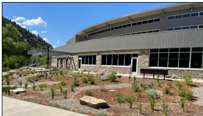
Santa Rita Water Reclamation Facility's Demonstration Gardens incorporate many plants native to Colorado and the Southwest. © Bill LeMaire
