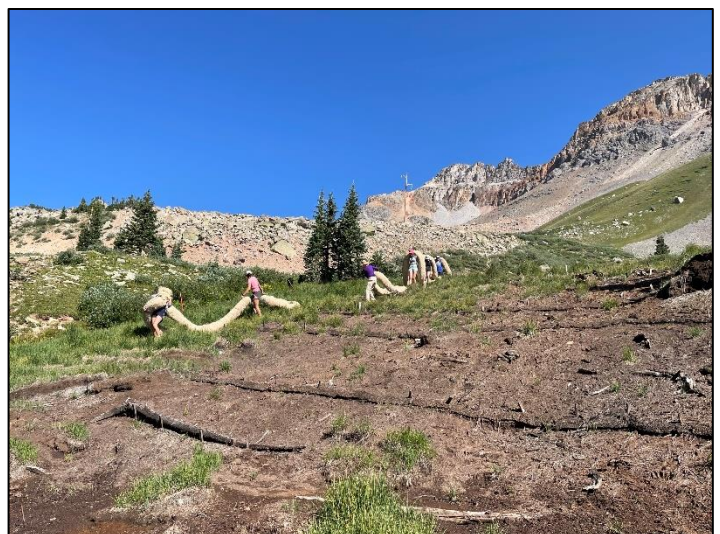
Volunteers install erosion control materials at Ophir Fen. © Amanda Kuenzi
