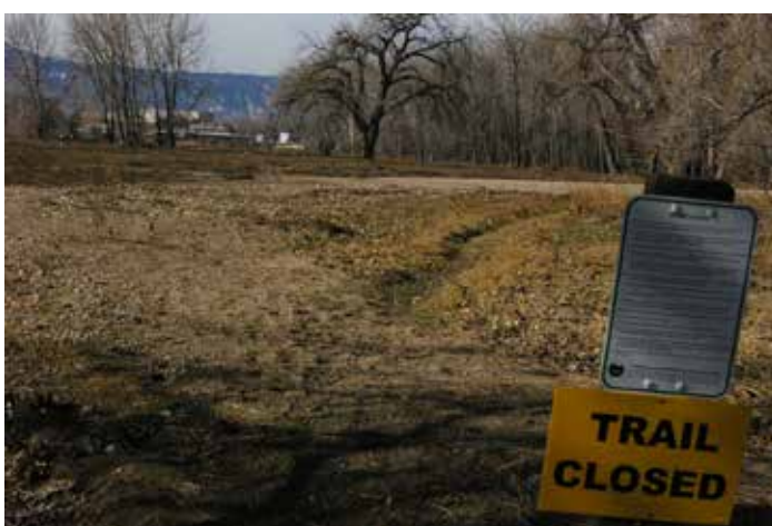
South Boulder Creek Scouring
